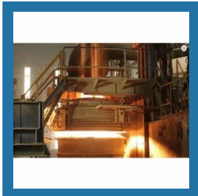
Electrotherm Laddle Refining Furnace
