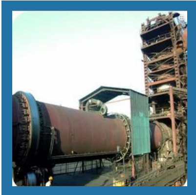
Rotary Kiln Coal Based DRI Plant
